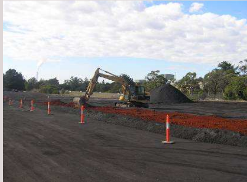
Blending trials of filtercake & mill scale
